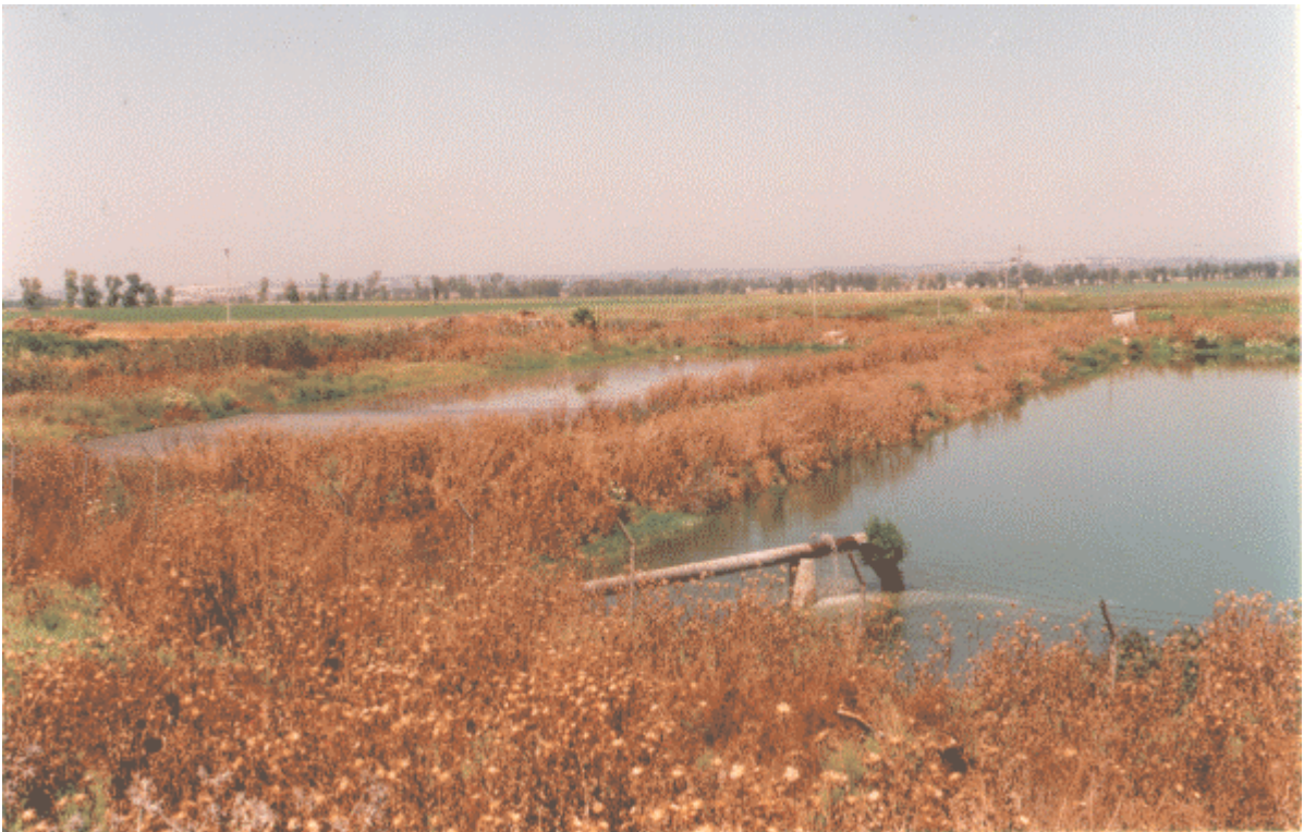
Photo 1: Wastewater Treatment Plant for Tulkarm City
