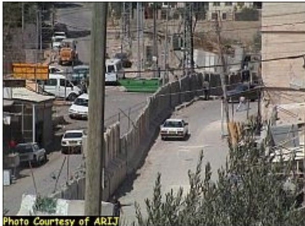
Photo Courtesy of ARIJ The existing concrete Wall in Abu Dis city.
