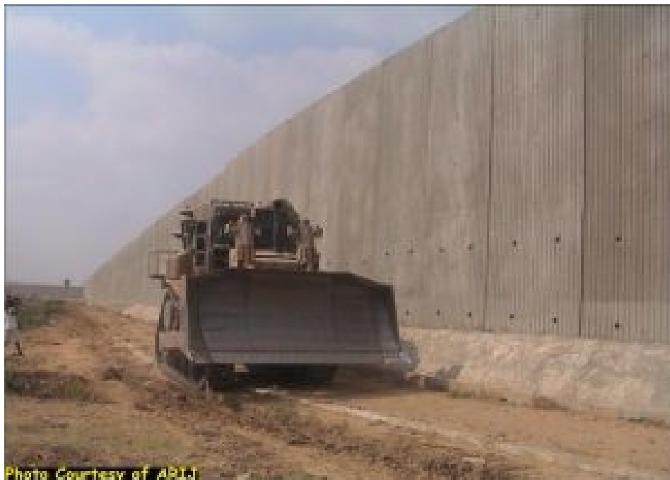
Photo 3: The Segregation Wall 6-8 meters high west of Qalqiliya city, 2003
