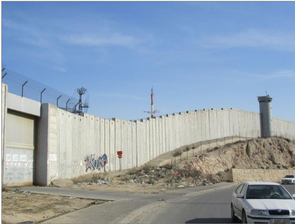
Photo 1: The Segregation Wall
