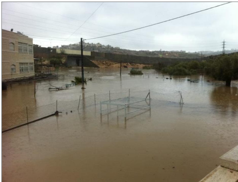
Photo 7: Blocked drainage causing water and wastewater flooding of residential areas and agricultural lands
