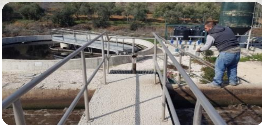
Work during operation and maintenance of Wadi Al Arroub WWTP
