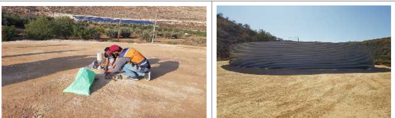
Site Sludge Dewatering arrangements and under construction water reuse reservoir
